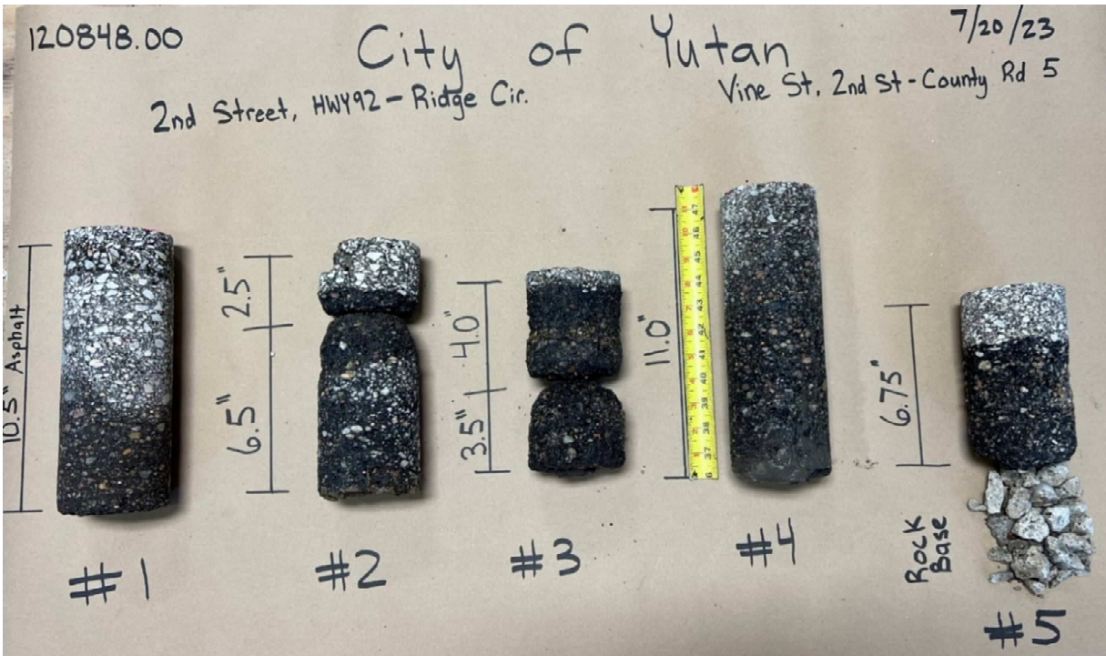
FIGURE 4.1: PAVEMENT CORE PHOTOS #1 - #5
